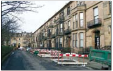
Typical rehabilitation works
