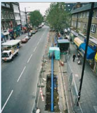
Typical watermain replacement
