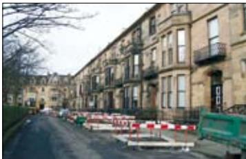
Typical rehabilitation works
