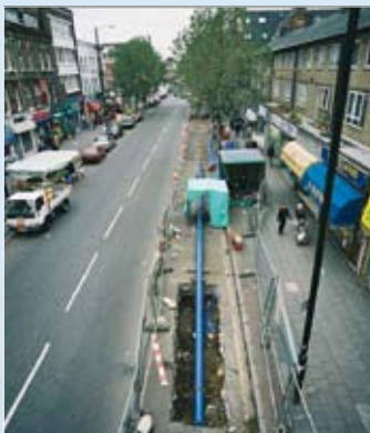
Typical watermain replacement
