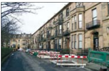
Typical rehabilitation works
