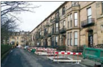
Typical rehabilitation works
