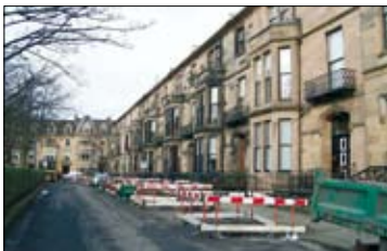
Typical rehabilitation works
